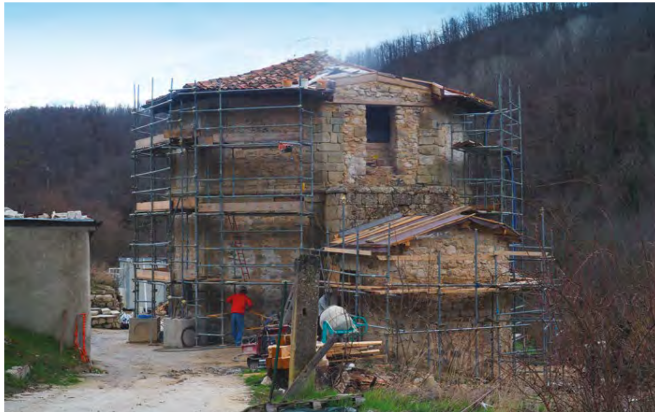
Below: the restoration of the Oratorio di Santa Maria del Sole, Capodacqua (Ascoli Piceno). Opposite, above: two horologists maintaining the antique clocks
